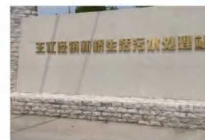
Wangjiangjing Town Xinqiao Domestic Sewage Treatment Station
