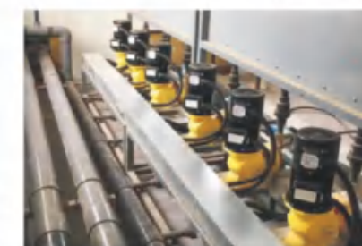
Hohhot Xinxinban Sewage Treatment Plant Expansion, upgrading and renovation project, with a processing scale of 200,000 tons per day
