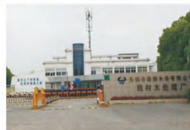
Wuxi High-tech Water Co., Ltd. Yingcun Water Treatment Plant The design scale is 210,000 cubic meters per day, and the initial daily processing scale reaches 50,000 cubic meters per day
