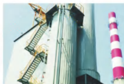
Hangzhou Hanglian Thermal Power
